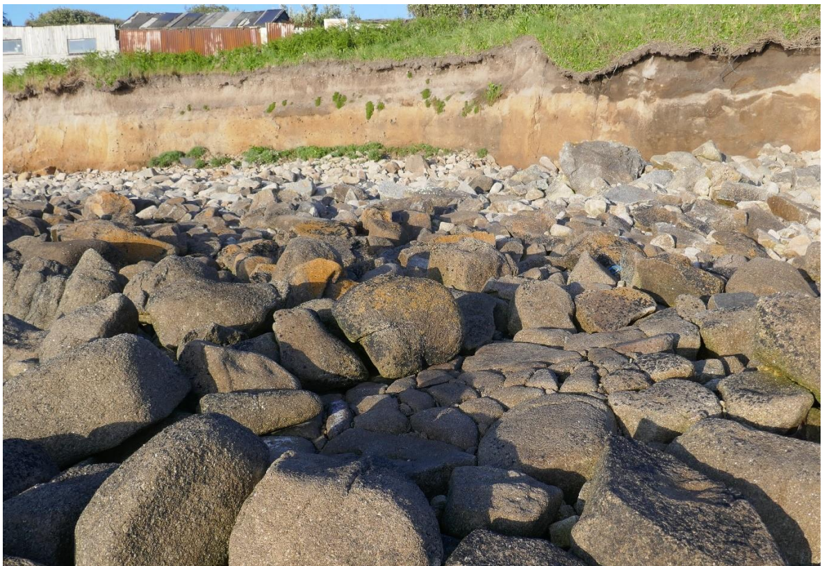
Fig 94 The mouth of a paved slip, with the base of sea front walling flanking it, at Porthcressa Brow, where the low cliff of ram (periglacial head) is continually eroding.
